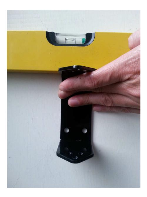
4. Marking 4 dots with pen through frame hole and drill the 4 holes at that dots by automation screw driver.
